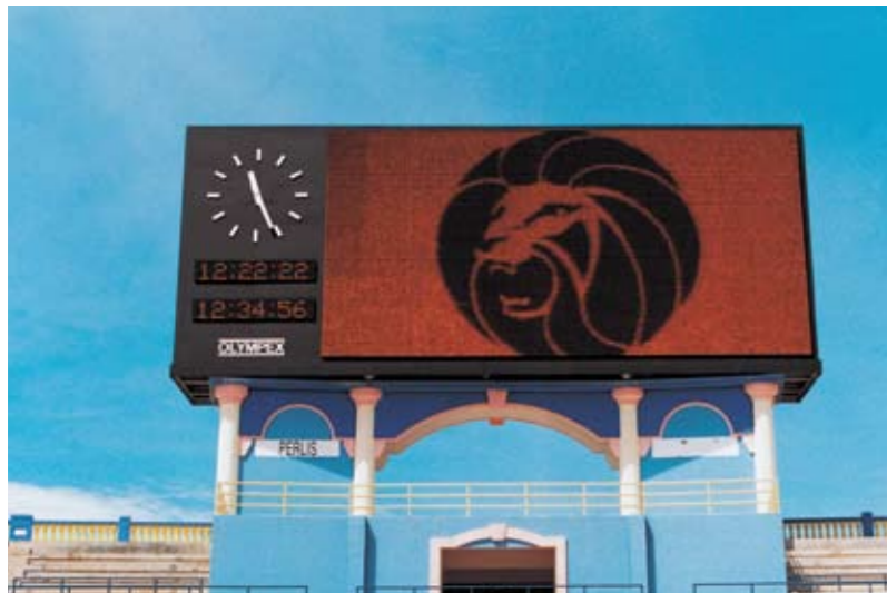
Shah Alam Stadium, Malaysia
