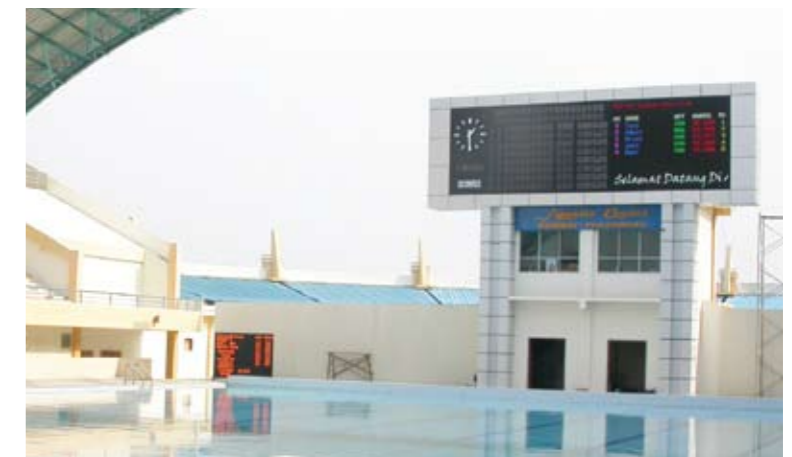
Rumbai Swimming Stadium, Indonesia
