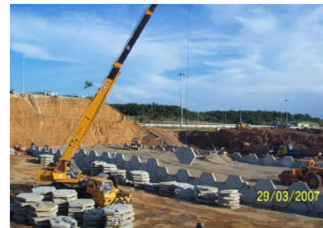
Panel installation and backfilling work is implemented simultaneously
